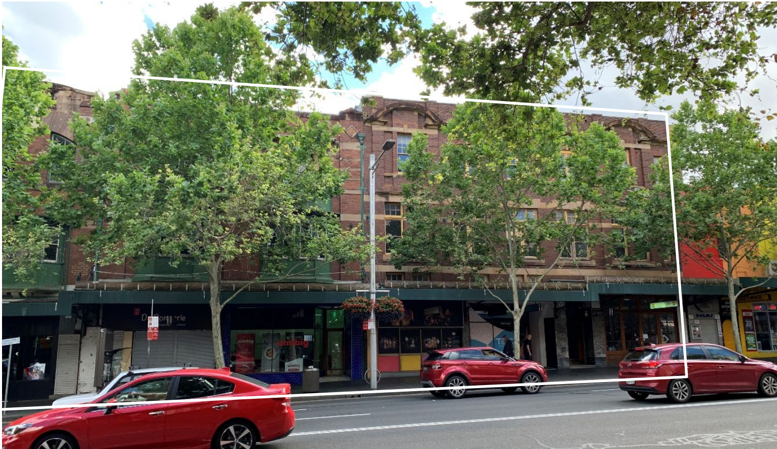
site viewed from Oxford Street
